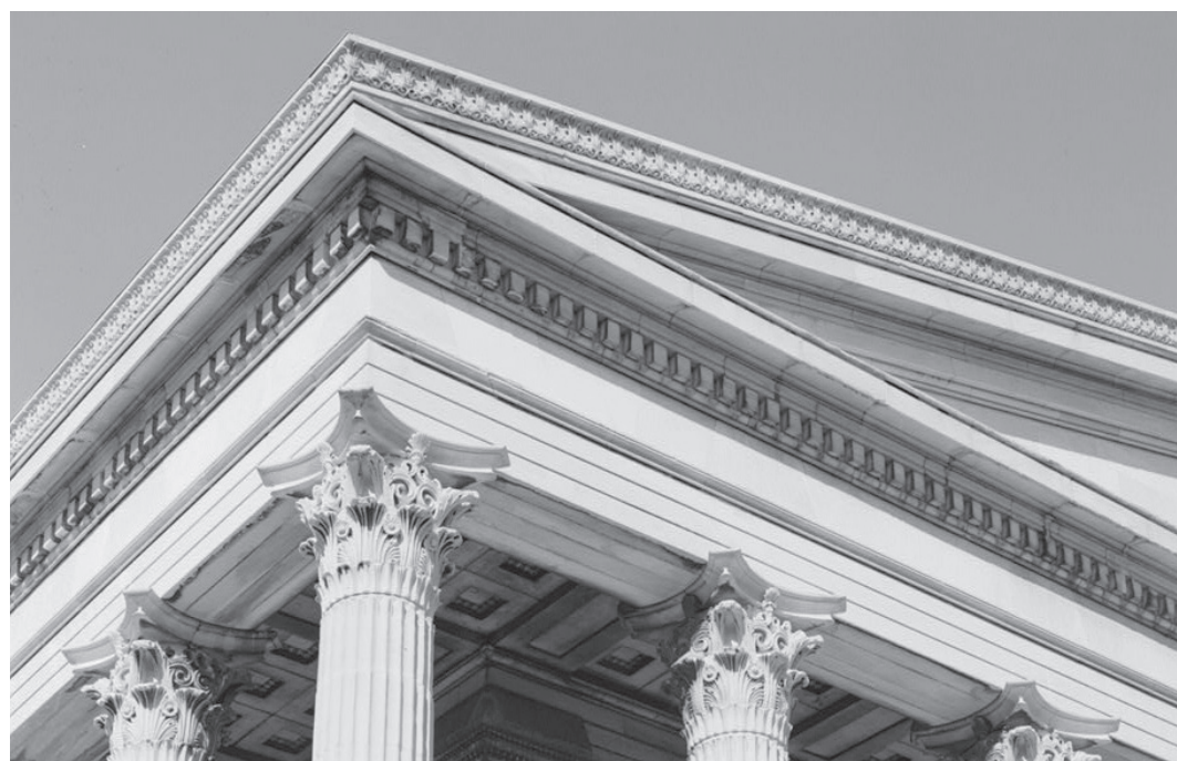
Fig. 78 - Historic American Buildings Survey, Girard College, Joseph E. B. Elliott, Jack E. Boucher, après 1933, photographie noir et blanc, Library of Congress (Washington, D.C.), HABS PA-1731
