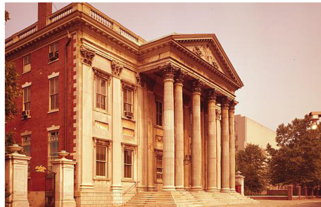
Fig. 27 - Historic American Buildings Survey, First Bank of the United States, 120 South Third Street, Philadelphia, après 1933, photographie noir et blanc, Library of Congress (Washington, D.C.), HABS PA-1417-6.
