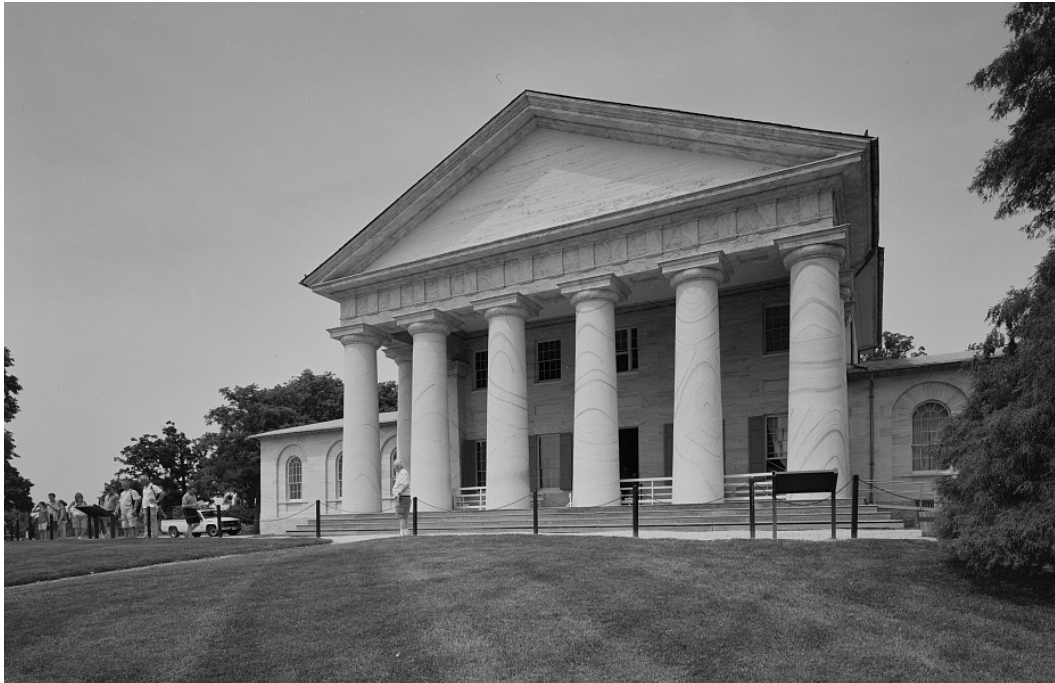
Fig. 31 - Historic American Buildings Survey, Arlington House, The Robert E. Lee Memorial Custis-Lee Mansion Robert E. Lee House, après 1933, photographie noir et blanc, Library of Congress (Washington, D.C.), HABS VA-443
